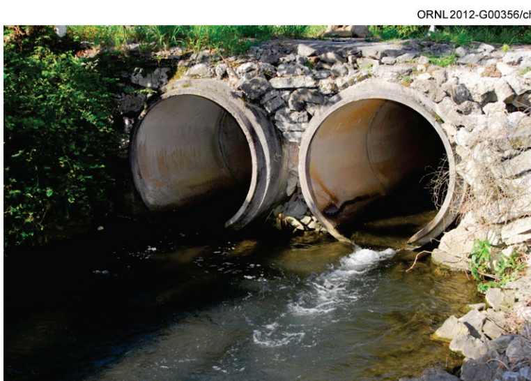
Fig. 4.46. Contaminated storm sewers were the primary source of mercury contamination in Poplar Creek.
