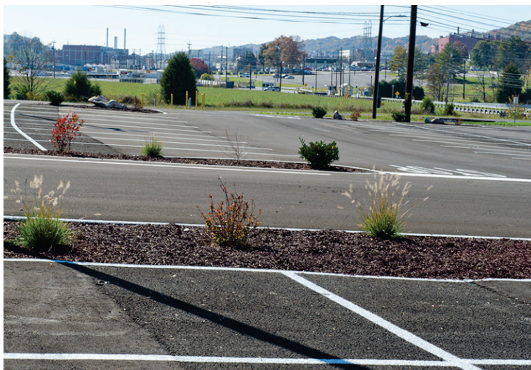
Fig. 4.15. Permeable pavement and native plantings contribute to Energy Independence and Security Act Section 438 requirements. (Source: Kathy Fahey, Y-12 Photography)
